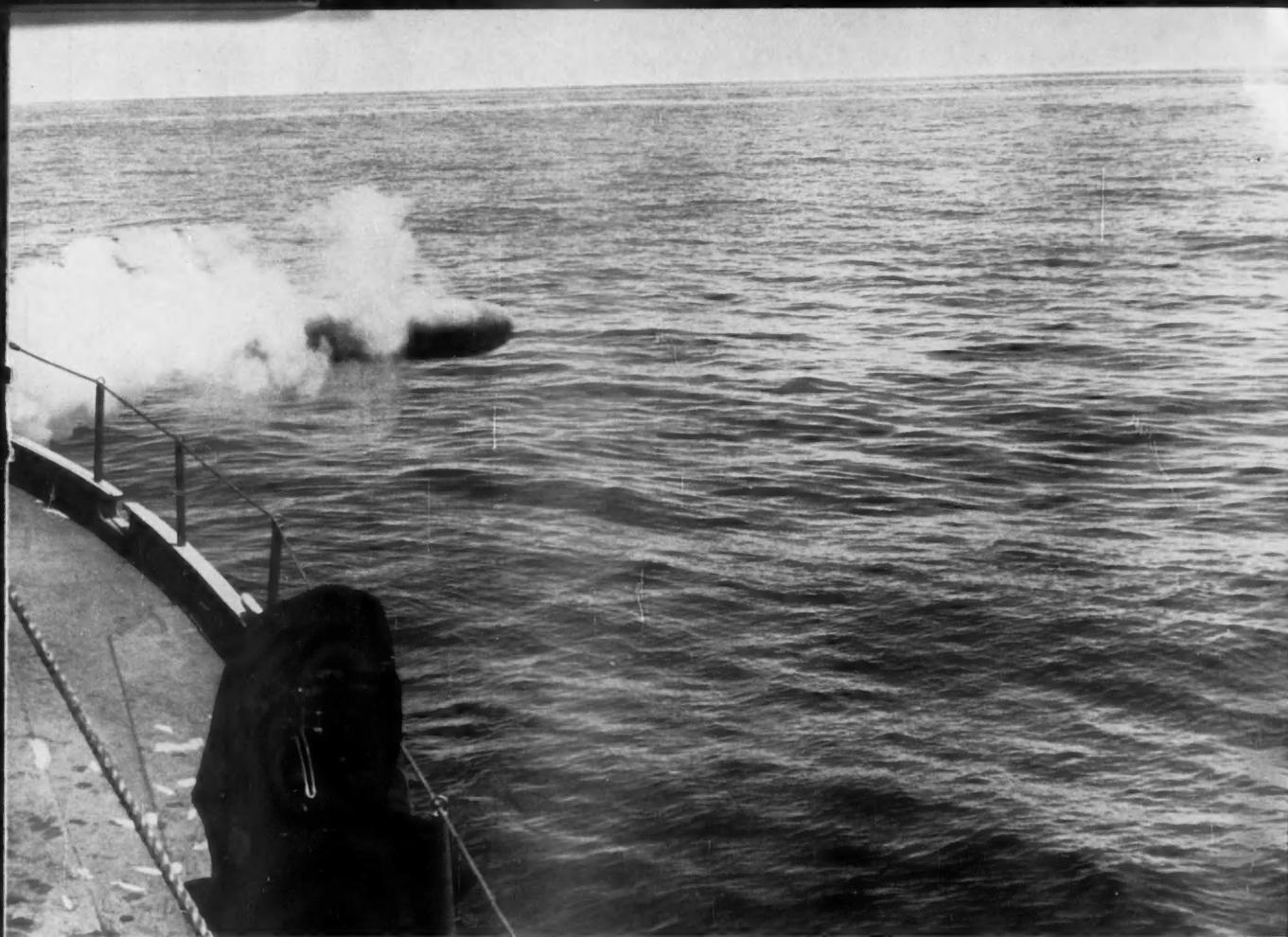
torpedo leaves deck launching tube of test ship to seek out target submarine. The torpedo is recognized as the Navy's pioneer guided missile.
