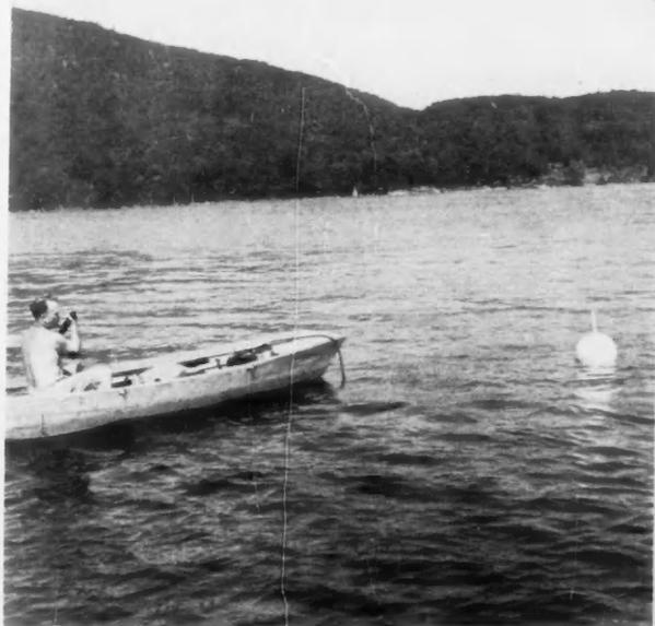
the water on an A-shaped frame that was supported by an 18-foot motor boat. The target: a pipe ring 10 feet in diameter suspended underwater from a buoy. Air pumped into a rubber hose peppered with holes that surrounded the ring sent up a cloud of bubbles that made an effective reflector for the sound waves sent from the transducer. By August the cry was, "We can sink any submarine in Lake George."
