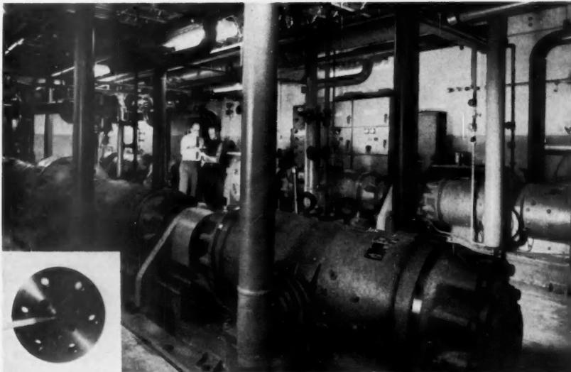
**VACUUM PUMPS** for helium tunnel fill an entire room and maintain a vacuum in the test section of the tunnel. Helium flows through a 1/10-inch orifice (inset).
