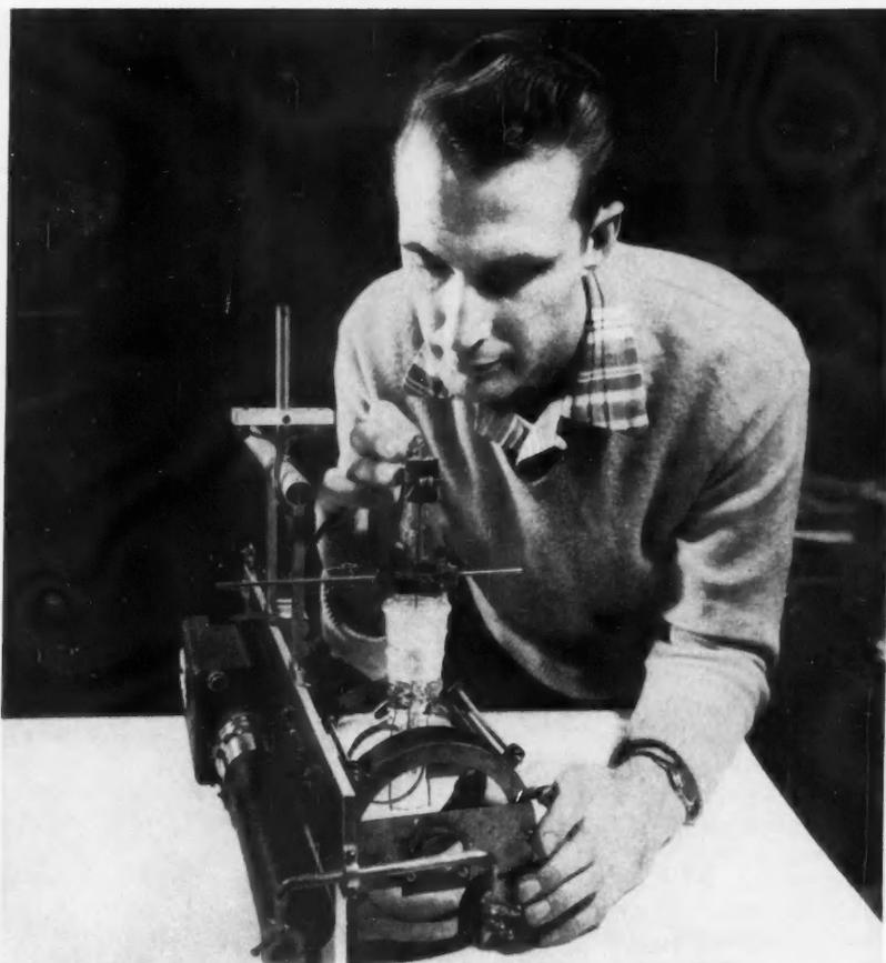
**MOVIE CAMERA**, light source, and glass cylinder attached to an aluminum supporting plate are used in a project to find out how fire burns in the absence of gravity.
