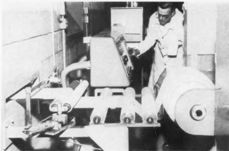
**RAW POLYETHYLENE** streams through 2-foot protective wall and beneath a million-volt electron generator for polymerization by cathode ray, during developmental production run.
