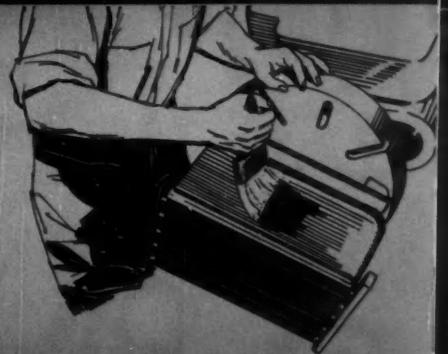
**IMPROVED BONDED FIELD POLES** for low-speed synchronous motors. Bonding technique continually advanced in large motor construction since 1938 inception.
