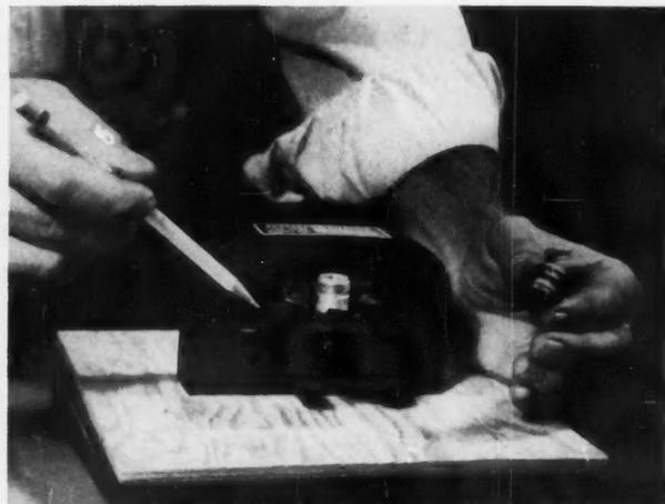
**COMPLEX IN STRUCTURE**, voltage-tunable magnetrons are supplied as package equipment, complete with permanent magnet and electron circuitry. Three VTM packages comprise (left to right) a low-power low-noise unit with a milliwatt output in the 2350 to 3100 mc range; a high-power narrow-band unit with a 10-watt output between 2900 and 3100 mc; and a general-purpose unit with minimum output of 2 watts in the 2200 to 3850 mc range. Pencil locates the VTM.
