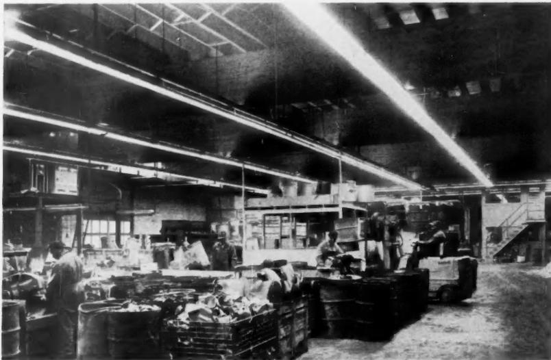
**POWER GROOVE UP-LIGHTS** supplement ceiling fixtures in the General Iron & Metal Corporation, Chicago, and aid workers to distinguish between colors in sorting salvaged metals.
