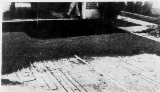
**BLACKTOP INSTALLATION** has 8-foot deep apron-wide cable arrangement tapering to 1½ feet for wheel tracks.
