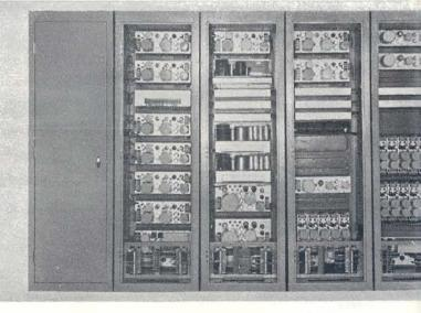
Actually the WSOY speech equipment is not all shown in these photographs as the complete equipment consisted of eight racks of apparatus and two custom design horseshoe type control desks. This speech input system is considered one of the finest in the world with every facility provided for multi-studio operation, master control and dual operation in its finest sense of the word.
