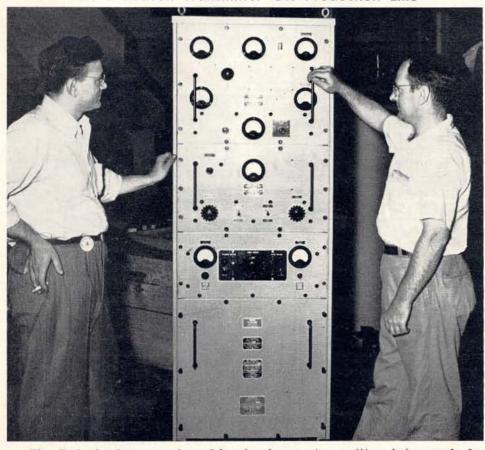
The first of a large number of homing beacon transmitters being made for the U.S. Government came off of the production lines the first week in June and is shown in the shipping department, ready for crating. These transmitters are 400-watt airport marker stations, both voice and code keyer modulated. The Continued on page 5)
