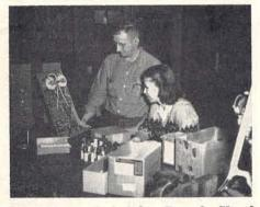
Art Brown is helping Beverly Shaul on the sub-assembly of an audio deck for a BC1-F transmitter.
