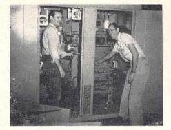
Jim Gibson and George Van De Boe are completing the final assembly of a BC1-F. Here the complete installation of all sub-assembly work as well as additional miscellaneous parts can be seen.
