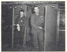
John Maxwell and Neal Middendorf are installing doors to complete cubicles after preliminary test has been made.
