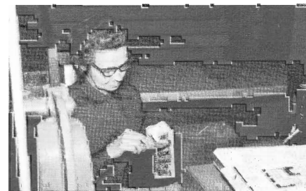
Georgia Vaughn completes the insertion of minute hardware parts onto a PC board.
