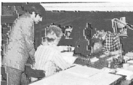
Bob Vaughan watches as Dianna Roate and Sharon Beedle inspect and touch-up the PC boards between the plating and etching procedure.
