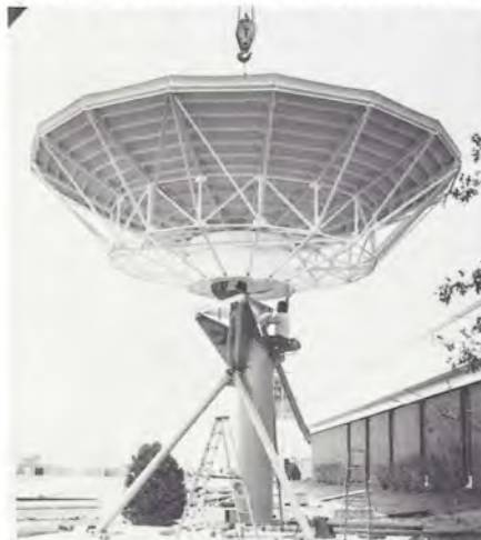
Once assembled, a crane lifted the reflector into position.
