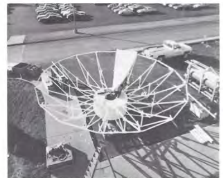
Assembly of reflector. Here the lacing is nearly complete and one reflector panel is being installed.
