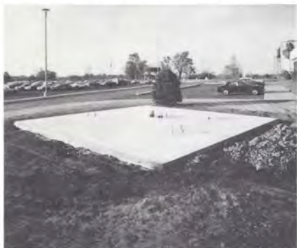
First step was the cement pad, a 27-cubic-yard foundation which was done by Shortridge Construction.
