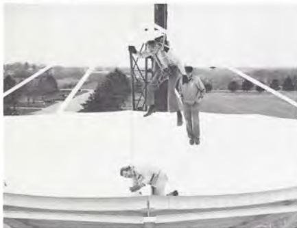
Suspended in air, Walt Beaver is assisting George Owens with alignment of the sub-reflector which had to be aligned two ways. For true alignment, Walt was held away from the assembly. Also pictured atop the reflector is Dale Willis.
