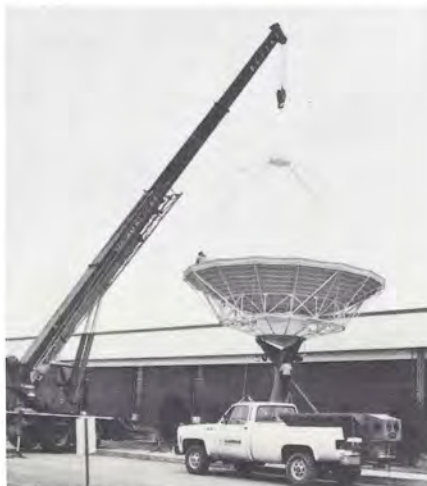
The crane was also used to place the subreflector on the reflector.
