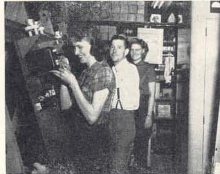
**Helen Spidle, Jim Medlin and Dorothy Smyser are shown mounting sub-assemblies on panels to be installed in a BC1-F transmitter.**
