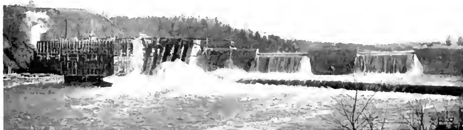
High water during construction, showing water passing over the unfinished sections of the dam spillway
