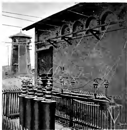
Fig. 7. Highland Park Substation, Charlotte, N. C., Showing Old Lightning Arrester Tower on left, G.E. Aluminum Cell Lightning Arrester and Horn Gaps in Foreground
