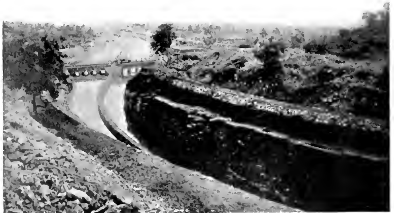
Fig. 4. Channels Through Rock Cutting
