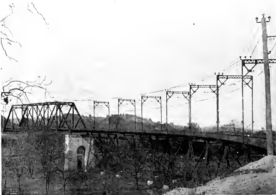
Fig. 8. 1200-Volt Overhead Line Construction on Steel Trestle, Pittsburg, Harmony, Butler and New Castle Railway, Pittsburg, Pa.
