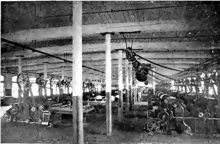
Fig. 2. Second Story of Picker Building Showing 200 H.P. Motors Suspended from Ceiling Rafters. White Oak Mills
