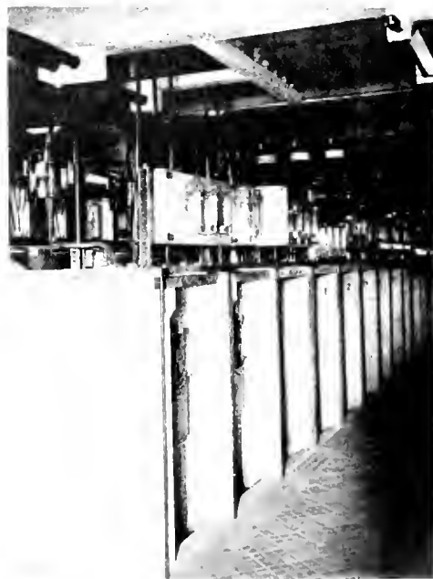
Fig. 12. Low Tension Switch Compartments
