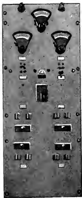
Fig. 11. Exciter Panel
