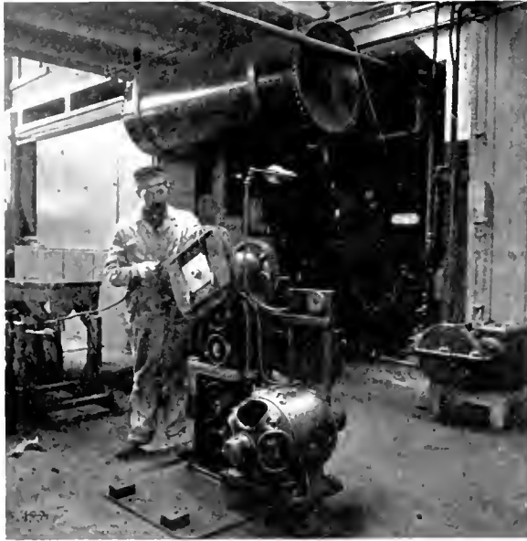
Winding a Field Coil in Repair Shop
