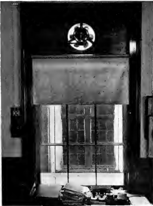
Installation of 12-Inch Alternating Current Ventilating Outfit
