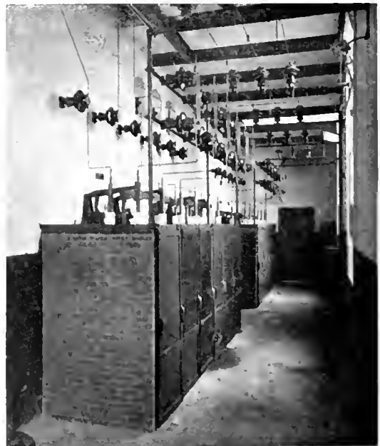
Fig. 8. High Tension Compartment Naval Academy Substation
