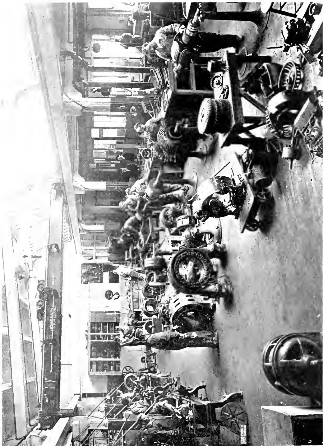
Armature Winding: General Motor and Armature Repairs. Repair Shop of the General Electric Company, Chicago
