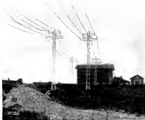
Fig. 5. 44,000 Volt Lines entering the Gastonia Substation
