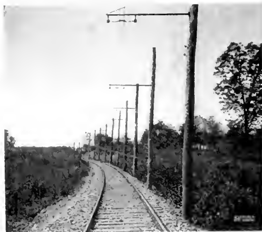
Fig. 7. 1200 Volt Direct Current Overhead Line Construction of the Pittsburg, Harmony, Butler and New Castle Railway, Pittsburg, Pa.
