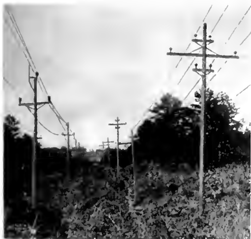
Fig. 2. Single and Twin Circuit Poles
