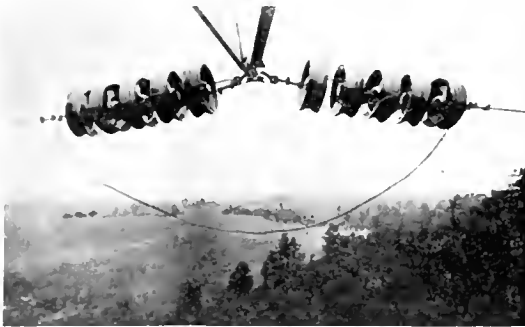
Fig. 10. High Voltage Strain Insulator
