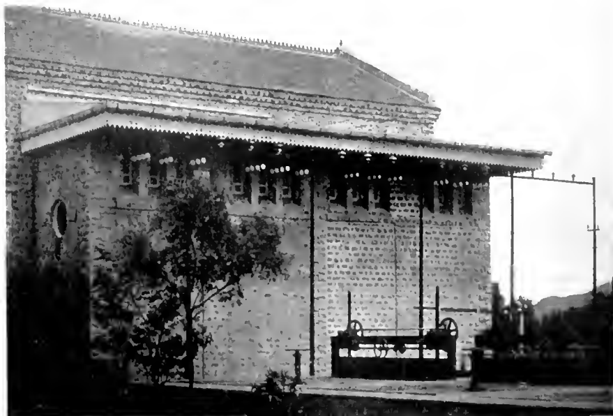
Fig. 14 High Tension Line Entrances to Step-Up Station
