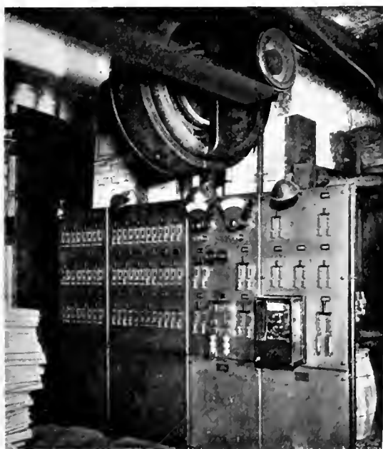
Fig. 1. 40 Kw. Generator and Main Switchboard
