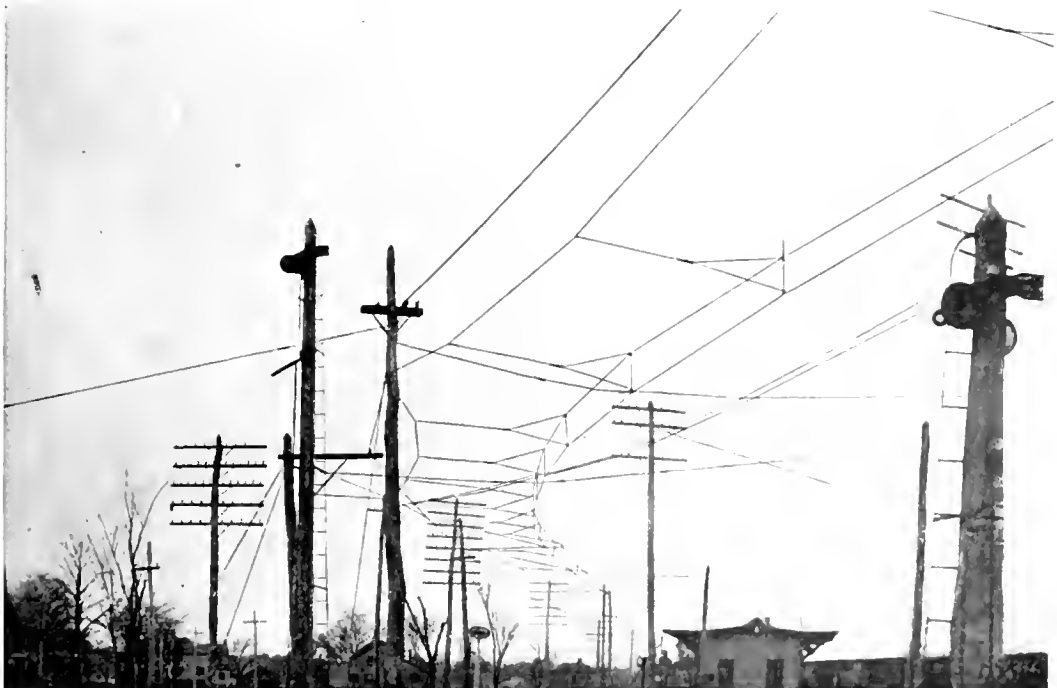
Fig 6 Pull-Off Construction
