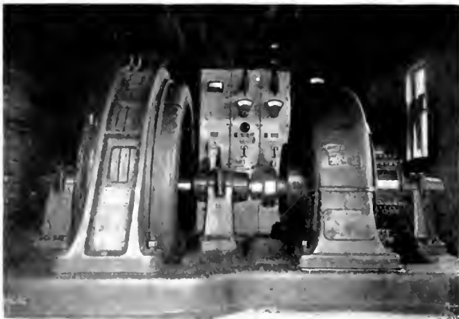
Motor-Generator in Substation
