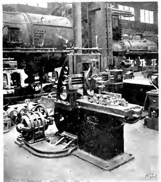
24 In. Planer Driven Through Gearing by 7\frac{1}{2} H.P., 750 R.P.M., 550 Volt, Form K Induction Motor
