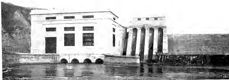
View looking up stream showing finished power house and sluice gate masonry
