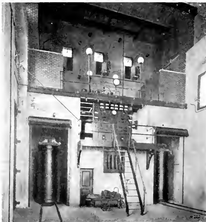
Interior view showing north end of power house and the general arrangement of transformer cells, switchboard, and high tension gallery
