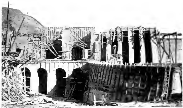
Tail race and sluice gate diverting wall during construction
