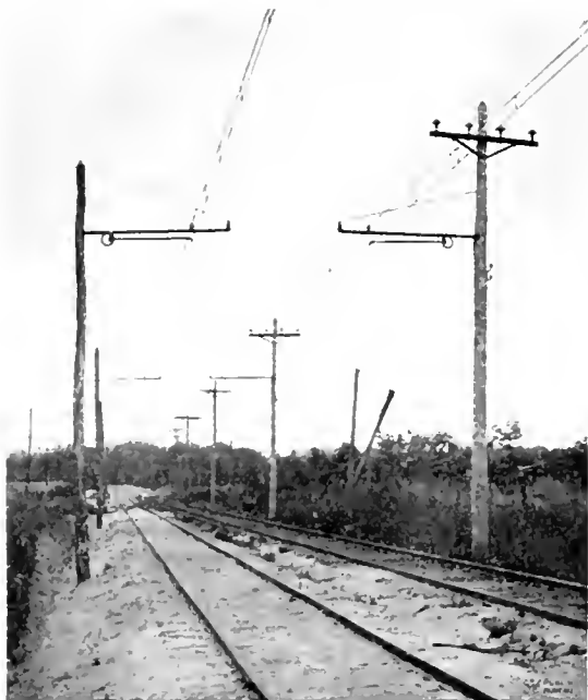
Fig. 6. Typical American Overhead 6600 Volt Single-phase Interurban Trolley Line, Baltimore and Annapolis Short Line, Annapolis, Md.
