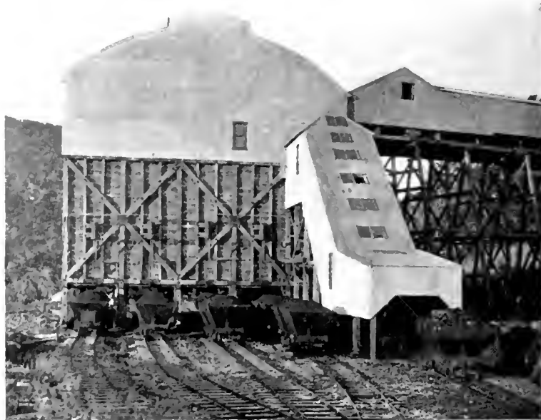
Tipple and Storage Bins, Showing Hydraulically Operated Doors
