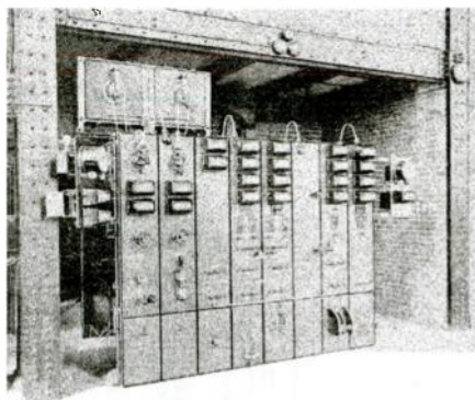
Fig. 11. Front Panels of Main Power Station Switchboard
