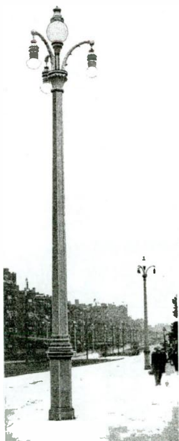
Fig. 2. One of the Poles Used for the Spectacular Illumination of Huntington Avenue, Carrying Four Colored Flame Arcs, the Upper One Pale Green, the Lower Three Light Rose Pink
