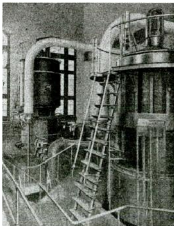
Fig. 6. One 800 Kw. and One 1500 Kw., 6000 Volt Three-Phase 25 Cycle, 1500 R.P.M. Vertical Shaft Turbo-Generators in Port Henry Power Station
