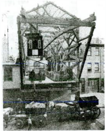
Fig. 8. Monorail Hoists Operated by One 75 H.P. and One 15 H.P. Motor. The United Engineering & Contracting Co., New York City
