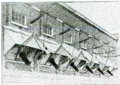
Fig. 5. 140,000 Wall Entrances at Zilwaukee Substation of Eastern Michigan Power Company
