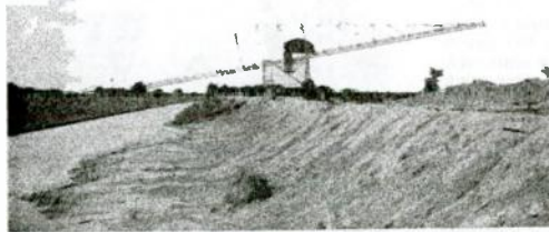
Fig. 7. Cantilever Crane Operating Drag Bucket made by Brown Hoisting Machinery Co. 225 H.P., 400 Volt Induction Motor. The United Engineering & Contracting Company, Barge Canal Contract No. 40, Lockport, N. Y.
