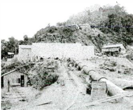
Fig. 4. Forebay 640 meters above Power House
