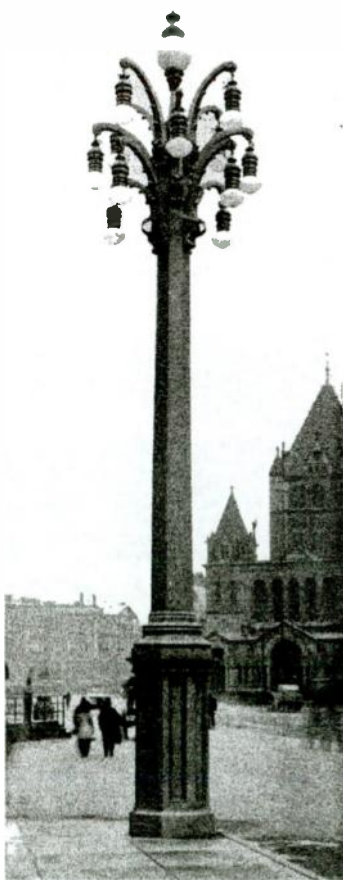
Fig. 3. One of the Special Pyrons Erected at the Ends of Huntington Avenue, 35 Feet High to the Upper Arc. Each Pyron Carries Thirteen Flame Arcs Colored Green and Pink
