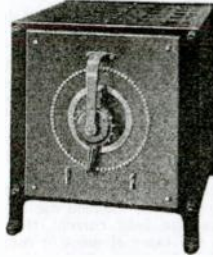
Fig. 2. Sprocket-operated Tube-type Rheostat
