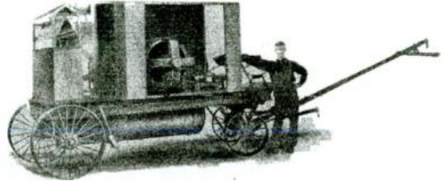
Fig. 4. 35 H.P., 500 Volt D-C. Motor Geared to Ingersoll-Rand 10x10 In. Portable Air Compressor, Havana, Cuba
