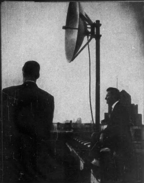
TERMINUS of microwave relay atop building in Newark, NJ. Antenna is only a few inches long.
