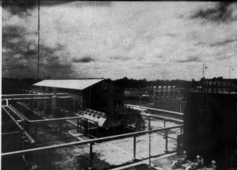
COMPRESSORS are located in stations spaced approximately 90 miles apart. The seven exhaust stacks at left connect to compressor-drive engines. Each station reports hourly to the chief dispatcher in the Houston office.
