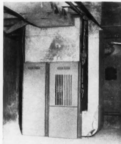
WATER-COOLED AND GAS-HEATED UNITS WORK SIDE BY SIDE TO KEEP THIS NORTHERN NEW JERSEY HOME COMFORTABLE YEAR ROUND.
