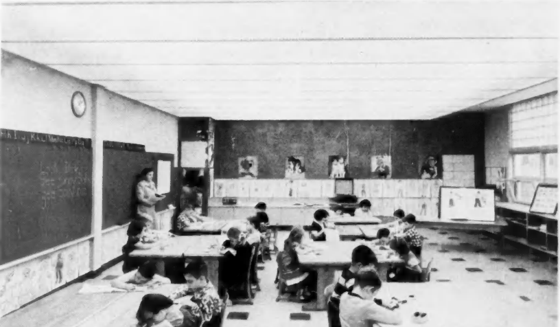
LUMINOUS PLASTICS CEILINGS INDICATE A TREND TOWARD COMPLETELY BUILT-IN LIGHTING.
