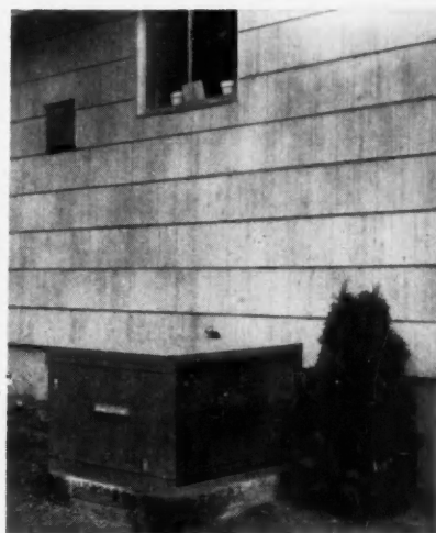
AIR-COOLED CONDENSER REDUCES WATER BILL.
