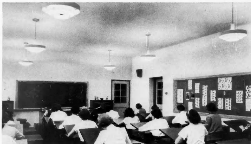
HIGH VISIBILITY IS OBTAINED WITH SILVERED-BOWL INDIRECT INCANDESCENT LIGHTING.
