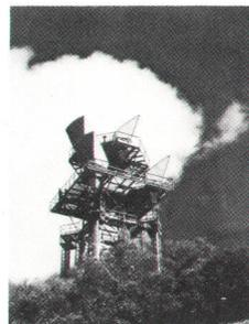
**Cover:** Keeping a microwave communications repeater—like the one shown on the front cover—operating at full efficiency means that the waveguide feedlines must be free of impedance discontinuities. Particularly disconcerting are multiple discontinuities, which degrade system performance
