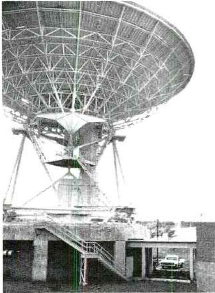
Figure 2. Antenna with track and wheel assembly - Palu, Hawaii Earth Station.
