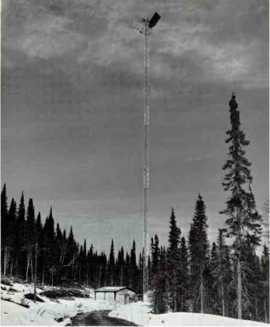
Figure 1. A "periscope" antenna system can provide path clearance without the expense and transmission impairments of a long section of waveguide.
