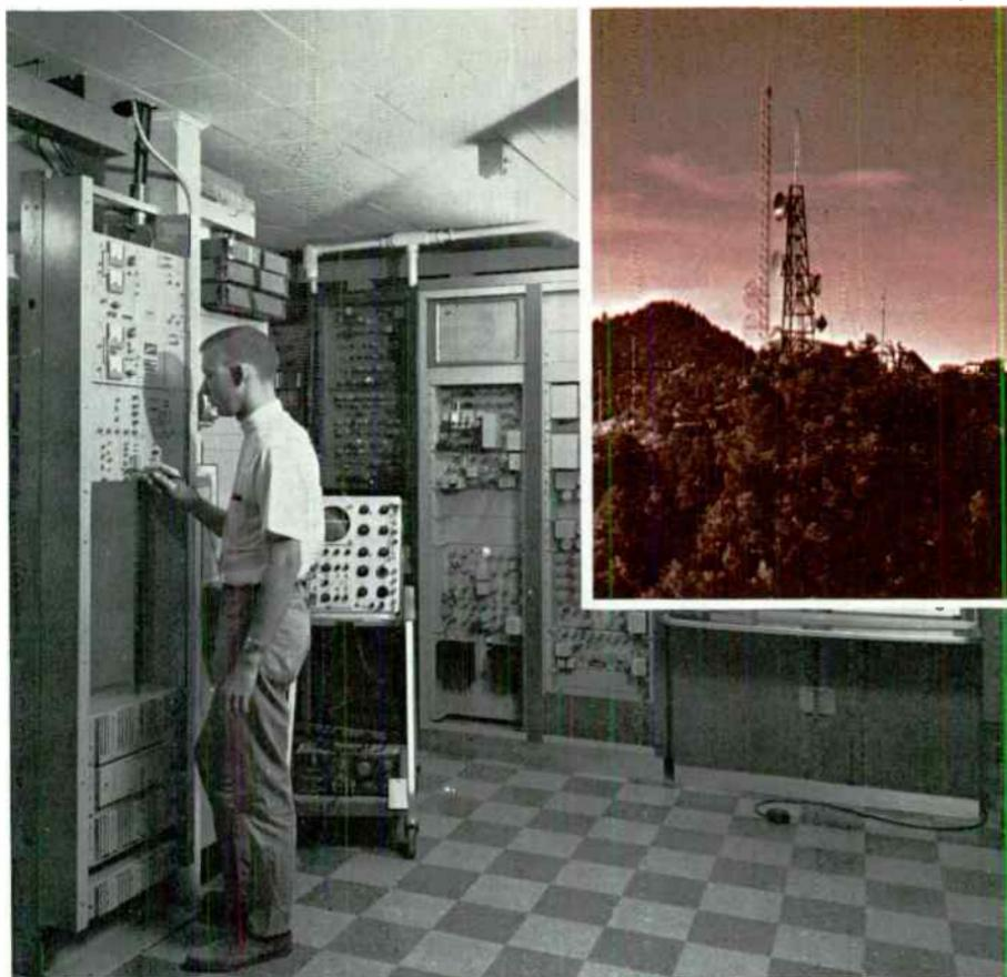
*Figure 4. Lenkurt 76TV microwave radio in typical installation. Repeater stations (inset) receive and retransmit signals.*
