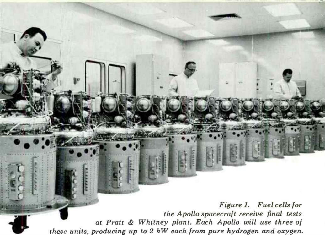
*Figure 1. Fuel cells for the Apollo spacecraft receive final tests at Pratt & Whitney plant. Each Apollo will use three of these units, producing up to 2 kW each from pure hydrogen and oxygen.*
