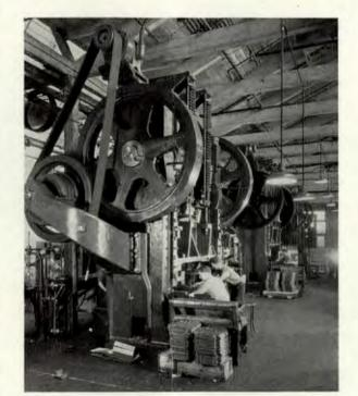
Fig. 2. Giant Double Crank Punch Presses, exerting 350 tons pressure, forming a sub-base for Philco Radio Chassis
