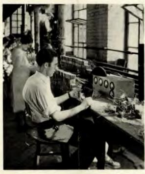
Fig. 7. Philco inspector testing completed By-Pass Condensers
