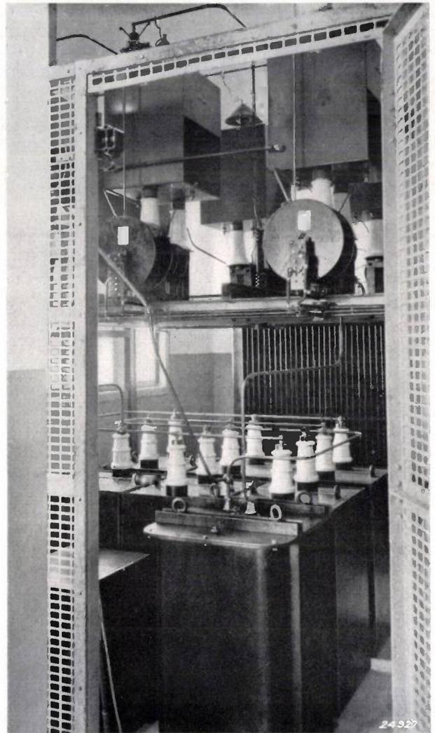
Fig. 22. The rectifier installation for the 60 kW stages. ]
