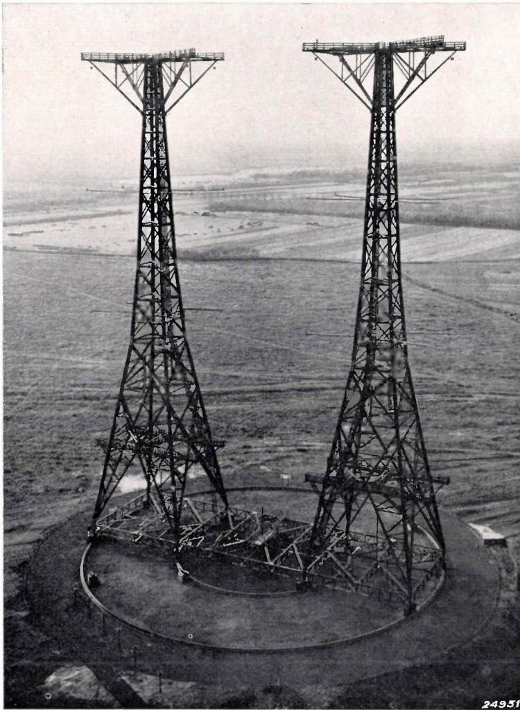
Fig. 6. The wooden towers of the rotating aerial.
