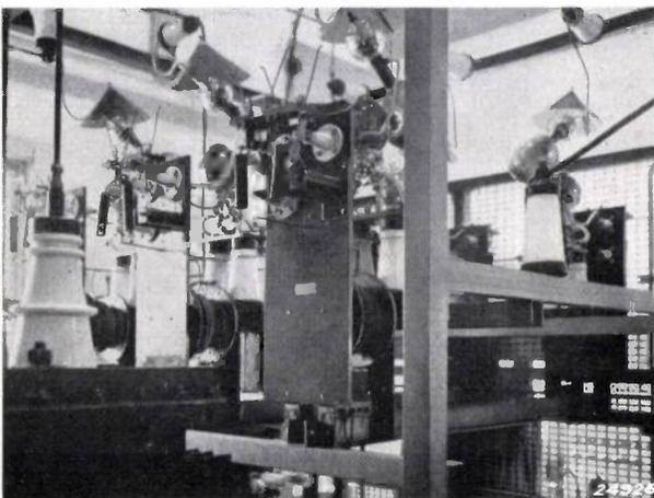
Fig. 21. The rectifiers D.C.G. 10/15 which feed the third section.
