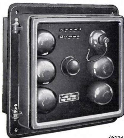
Fig. 4. Philips voltage regulator type 4142.
