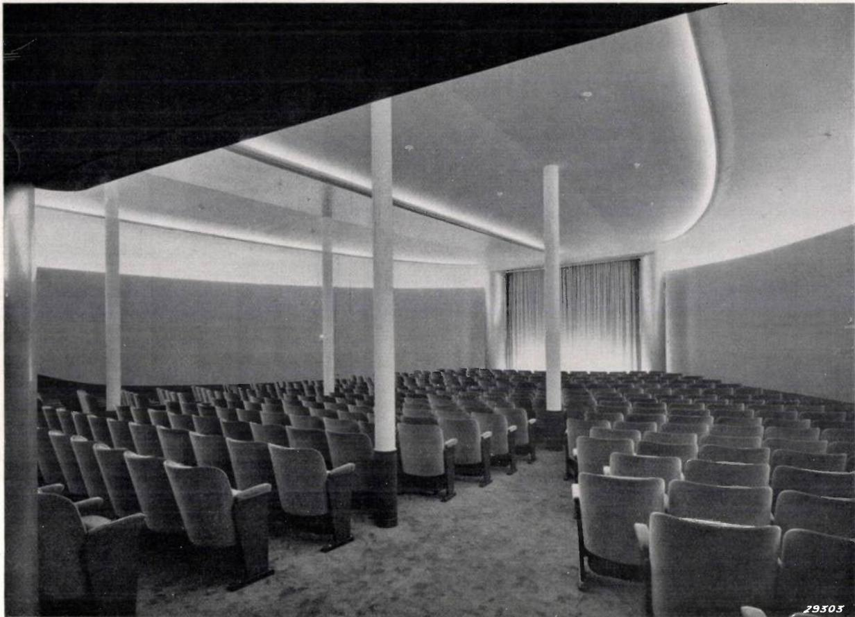
Fig. 6. Illumination of the theatre and cinema hall of the "Nieuw Amsterdam", which seats 350 persons. In order to lose nothing of the height the illumination had to be built into the walls and ceiling. A continuous line of tube lamps was installed along the three narrow bands where the slightly curved surfaces of the ceiling meet. In addition a light recess was made above the wine-red wainscoting, and equipped with a double row of tube lamps.
