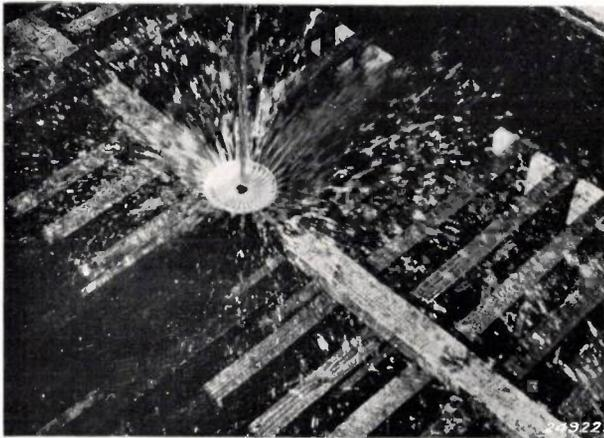
Fig. 17. The cooling water splashes against the wooden lattice-work of the cooling tower.
