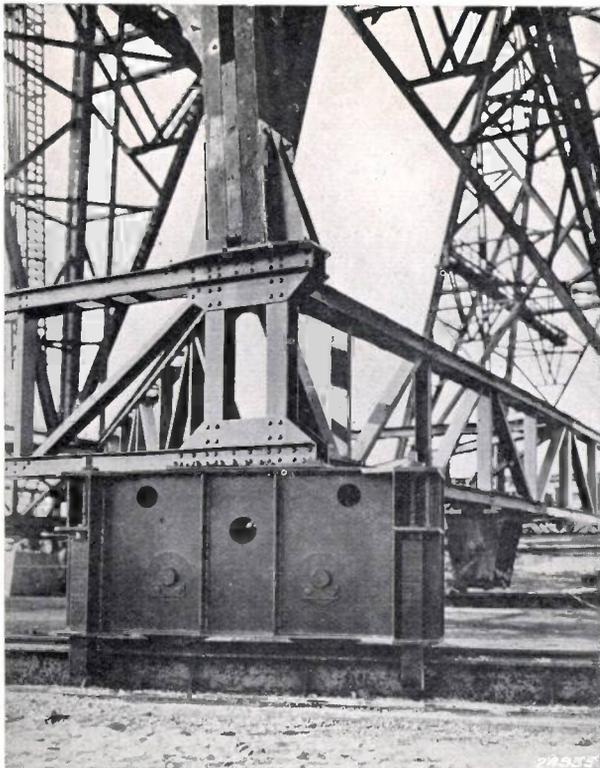
Fig. 4. Wheel boxes on the outer track.
