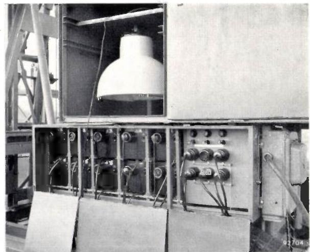
Fig. 3. A fitting mounted on its frame in the light-tight compartment on the trolley, where several fittings with lamps already burning can be stored. When changing a fitting, then, no time is lost waiting for the lamp to come up to temperature. Below the compartment can be seen the various ballasts needed for the lamps.
