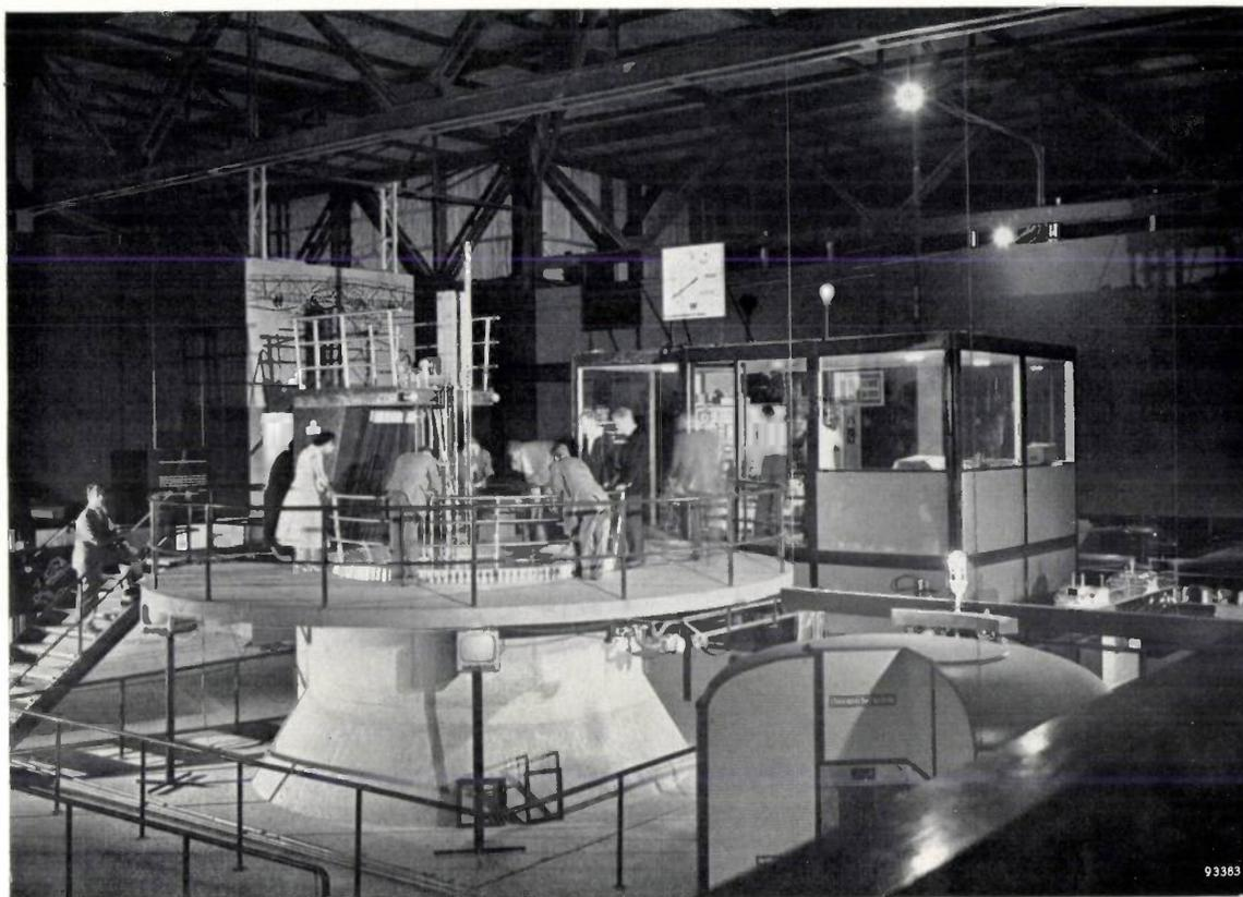
Fig. 1. Experimental nuclear reactor of the swimming-pool type at the exhibition "Het Atoom" in Amsterdam (Schiphol Airport). The photograph shows the upper part of the cylindrical tank, around which a platform has been fitted for visitors. The monitoring, control and safety equipment is installed in the cabin in the background.
