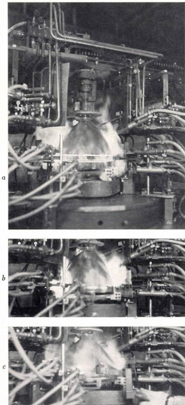
Fig. 10. A tube of the type shown in fig. 9 in the process of being sealed:
