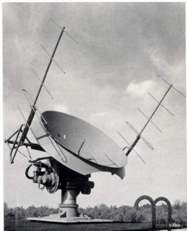
Fig. 3. The Yagi array transmitting the 50 kW interrogating pulses of 2 m waves is mounted on a common pedestal with the receiving aerial, a 5 ft diameter parabolic reflector with nutating dipole. They are automatically kept aligned on the balloon.
