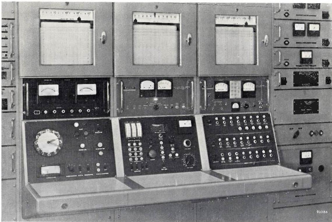
Fig. 7. Central section of console (cf. fig. 3). The three recorders above (from left to right) record respectively low neutron flux on a logarithmic scale ("log. C.R."), high neutron flux on a linear scale ("lin.  $N$ ") and high neutron flux on a logarithmic scale ("log.  $N$ "). Below the recorders are mounted the associated flux, period and power meters.
