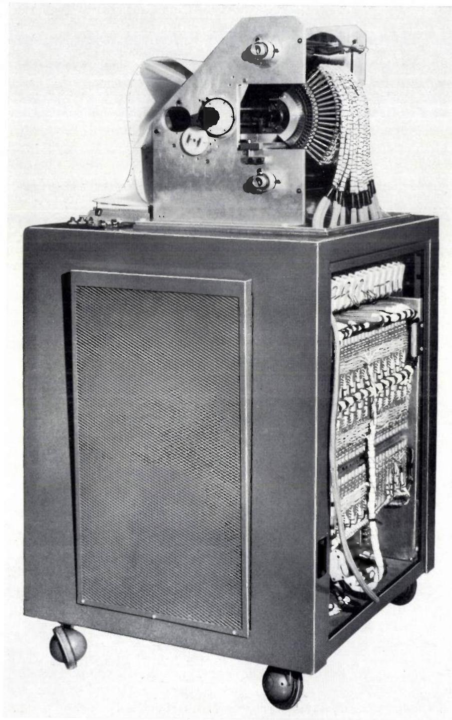
Fig. 18. Experimental model of the curve plotter.
