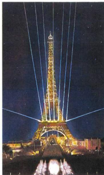
visitors climbing the tower in the evenings. The new system also cuts the electricity consumption by a half, and maintenance is now very much easier because a computer can identify breakdowns in any section of the system. The illumination is switched on automatically when the daylight level falls below 10 to 15 lux.
