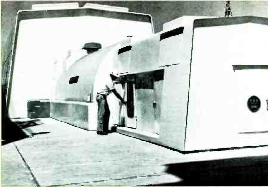
**1150-KW BRUSHLESS EXCITER** provides excitation power for 243-mva turbine generator at the Asheville Steam Electric Generating Plant of Carolina Power & Light Company.
