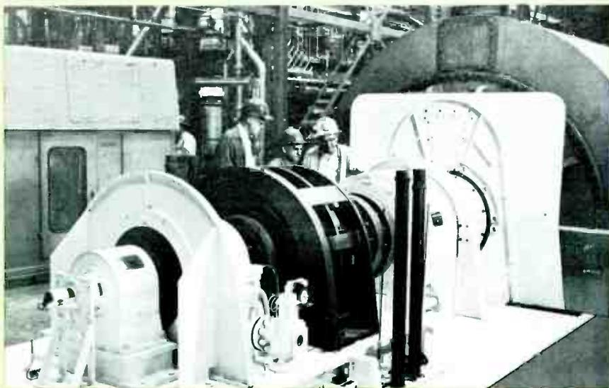
**TURBINE GENERATOR UNIT THREE** of West Penn Power Company's Mitchell Station is rated at 352 mva. The housing on the left end of the turbine generator contains the 1350-kw brushless excitation system. Brushless exciter system is shown with the housing removed (below). From left to right, major components are pilot exciter, ac exciter, fuse wheels, and diode wheel.
