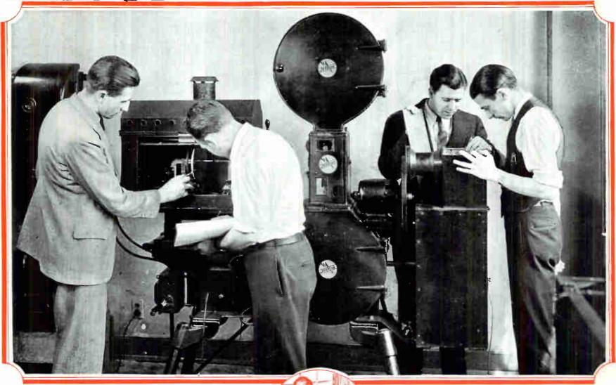
These men are receiving practical instruction on the operation. care and adjustment of the film scanning machine—a part of our Television transmitting equipment.
