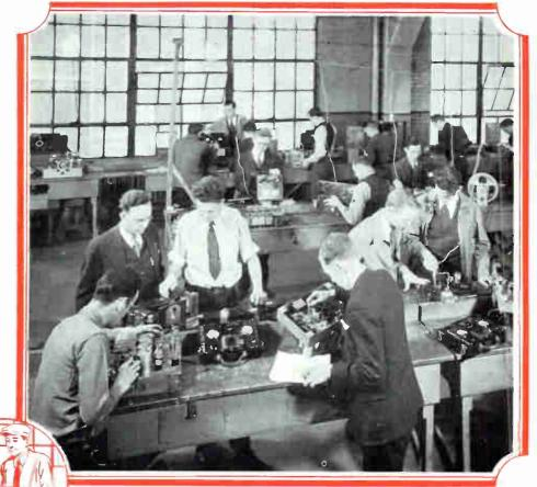
Students receiving instruction on use of modern set analyzers or trouble shooting kits. With this equipment it is easy to locate faults and defective parts in any type of set.
