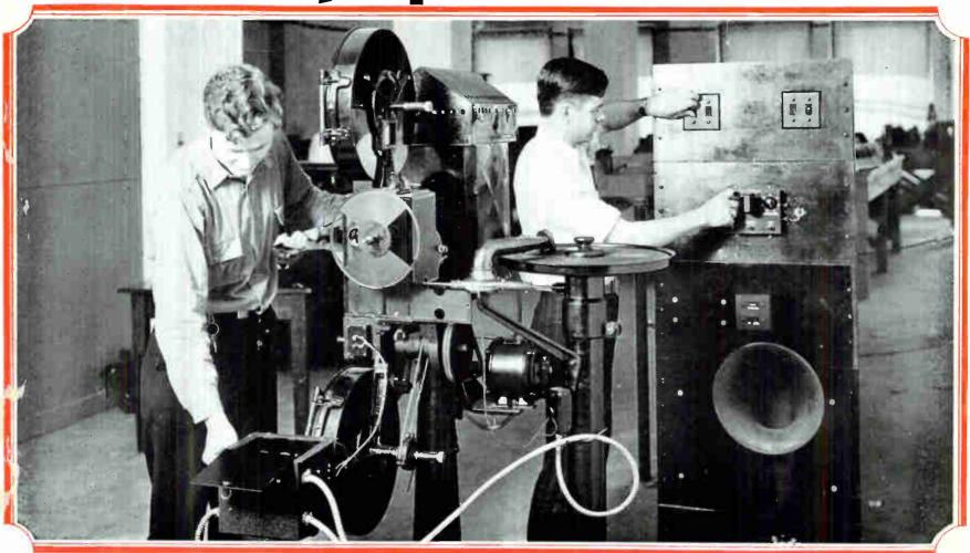
These students are learning the adjustment and care of sound equipment on talking picture machines. This machine is equipped to handle sound pictures of either the sound-on-film type or the film and record type.
