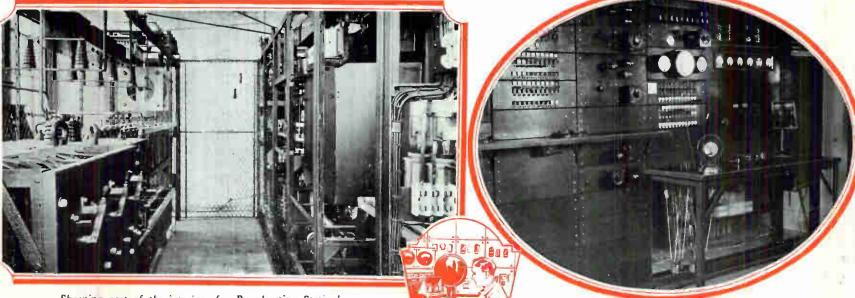
Showing part of the interior of a Broadcasting Station's transmitting coom. This is a 5 KW transmitter.
