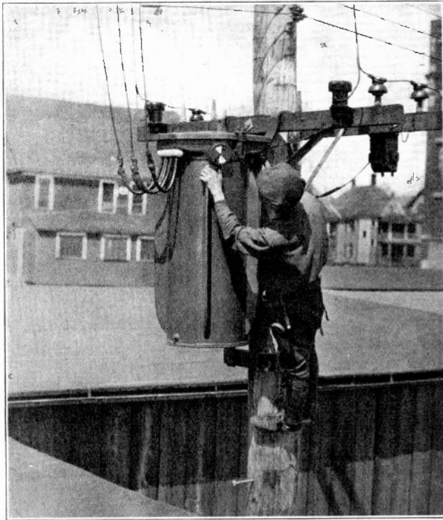
Fig. 124. This photo shows a pole type transformer and the method of making primary and secondary connections. Also note the thermometer temperature indicator near the hand of the electrician.
