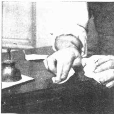
cloth which is then moistened with the rubbing oil. Dip the oily wad in the pumice powder and rub it into the filled-in scratch just as if you were sandpapering it. Be sure that you follow the grain of the wood. Finally polish the entire surface with furniture polish.
