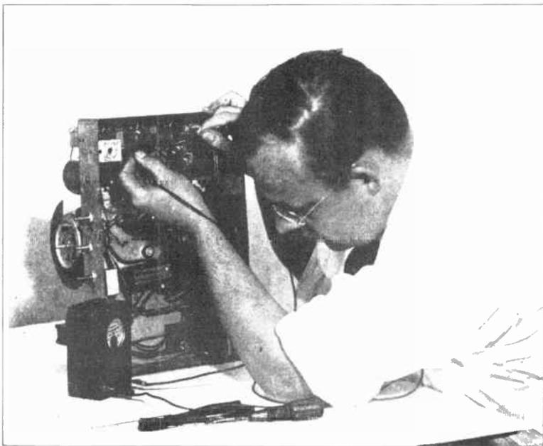
*Service man checking chassis with an ohmmeter*
