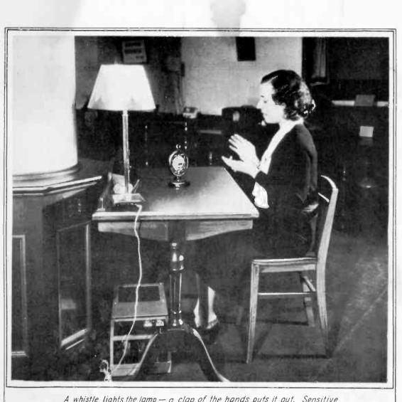
A whistle lights the lomp — a clap of the hands puts it out. Sensitive relays are used in this modern application of electromagnetism.
