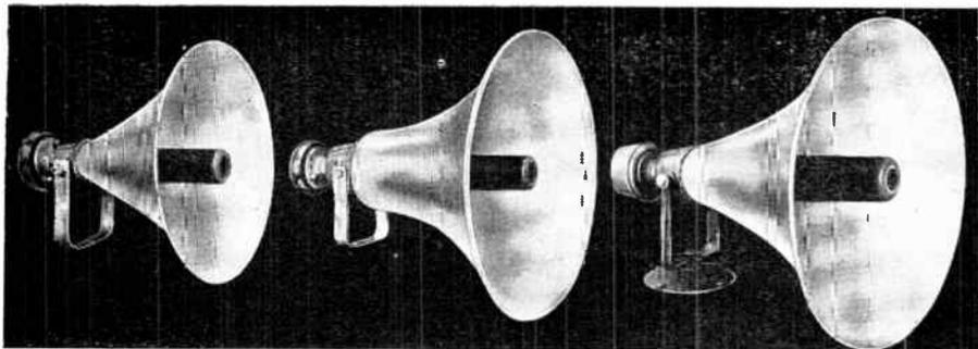
Here are shown three different sizes of speakers specially designed for outdoor use. They are of the dynamic reflex type. *Courtesy of Atlas Sound.*
