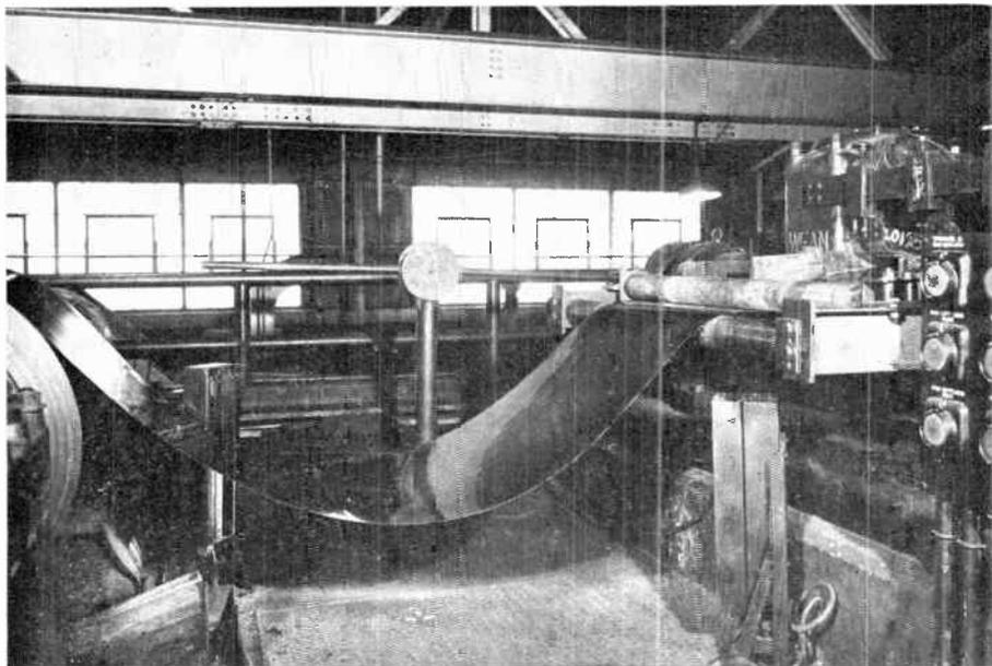
Here is shown an actual photoelectric installation for controlling the loop in a sheet of metal as it is rolled through the large rollers in a steel factory. The photocells are located at the left and the light source at the right. This installation is similar to the one illustrated in Fig. 9.
