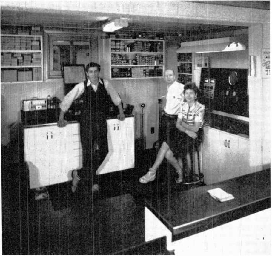
Here is a nice layout for the combination store-shop arrangement. There are two shop work benches one to the right along the wall with a convenient overhead fluorescent light. The other bench is along the rear wall and is used principally for heavy work, thus jars and shocks will not disturb the electrical instruments mounted on the panel. Note the use of shelves along the rear wall for spare parts and tubes. Courtesy of Sylvania.
