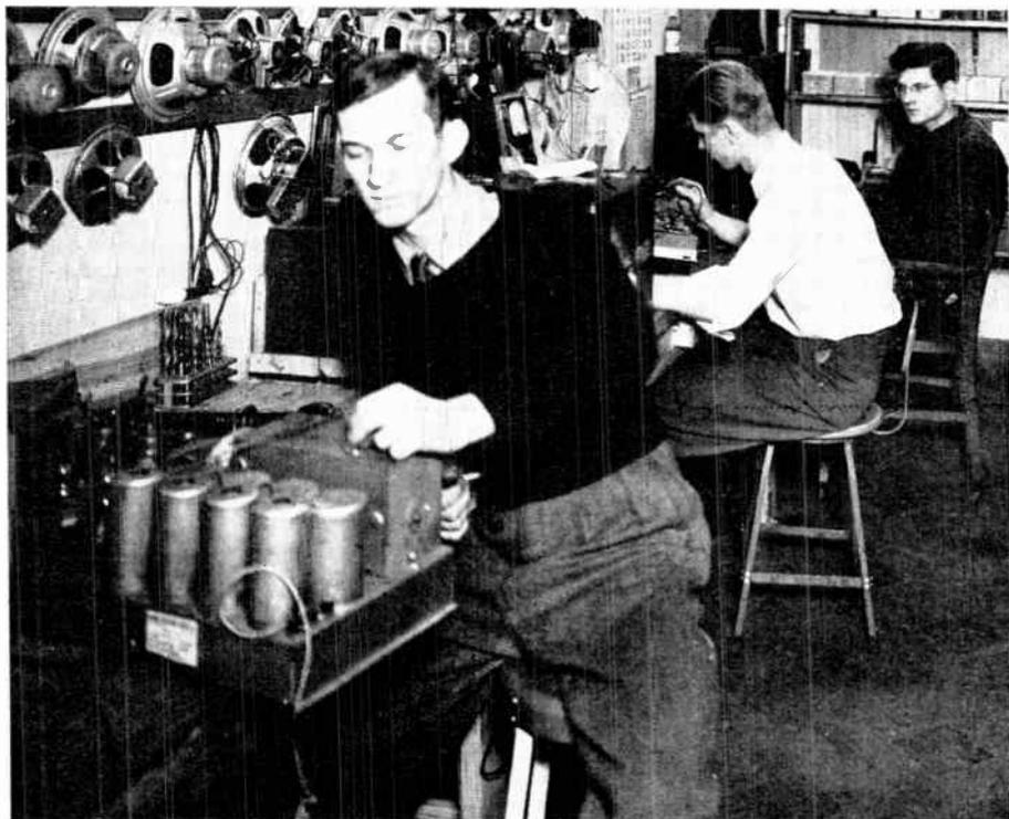
Here is a three man work bench with all test equipment portable so it can be moved about on the bench as needed. This is often desirable where several men must be working at once. In this case racks are often built along the back wall on which different pieces of test equipment may be conveniently placed. In this photo spare speakers are hung on nails above the workbench. Courtesy of Sylvania.
