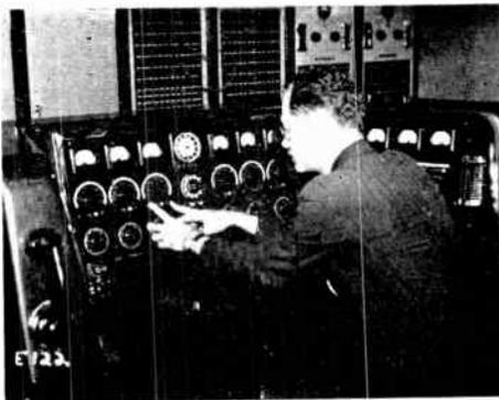
Automatic tuning systems are not confined to receiving circuits alone. They are used in many forms as transmitter controls. This view shows the control panel of a modern broadcast station employing several types of automatic controls which work in connection with relays.
