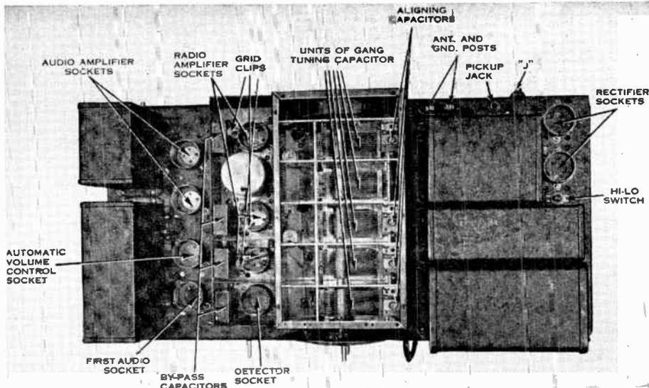
The above photo shows the layout of a TRF receiver which was in wide use at one time. Note the use of a five gang tuning condenser and the accompanying trimmer condensers which in this case are labelled aligning capacitors.
