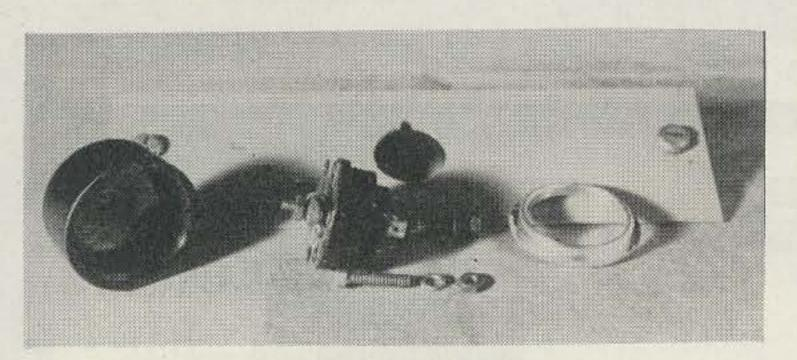
"Dismantled view of the T-17 switch showing mounting details."
