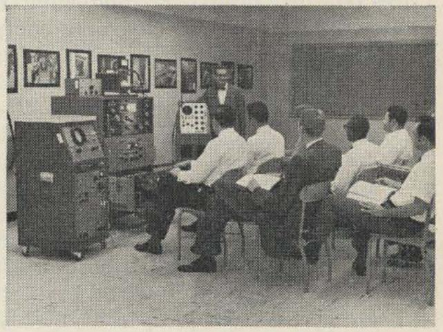
A recent class in session at the Nyack Transmitter Plant with TMC's GPT-750-E being tuned with the aid of TMC's PTE-3.
