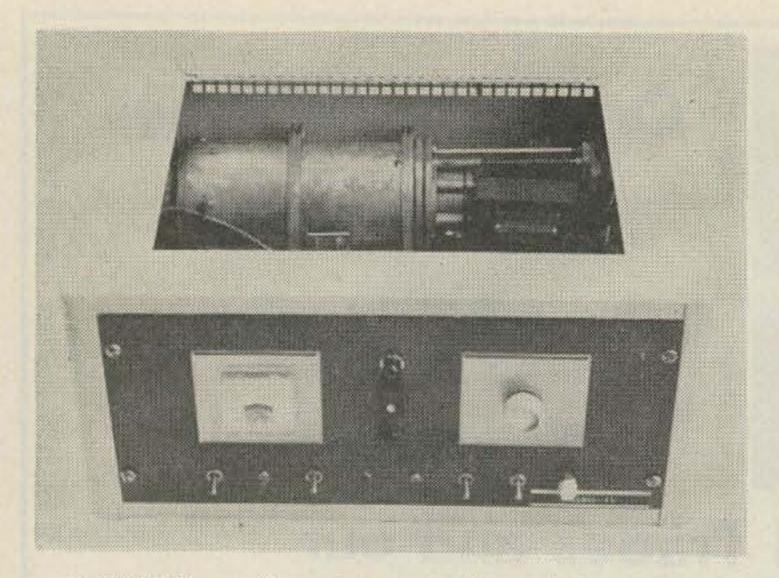
WA6BSL preferred to put the unit in a surplus cabinet and remote the switches to the front panel. Extra switches are for changing cameras.
