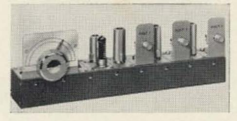
AOF VFO kit. 8-9 mc VFO for six and two meter transmitters.  $\frac{1}{2}$ watt output. AOF-89 includes VFO and buffer \$22. AOF-90 includes multiplier for six meter output \$29. AOF-91 includes multiplier for 6/2M output \$36. 6BH6 osc., OB-2 VR, 12BY7 buffer-amplifier & multipliers.
