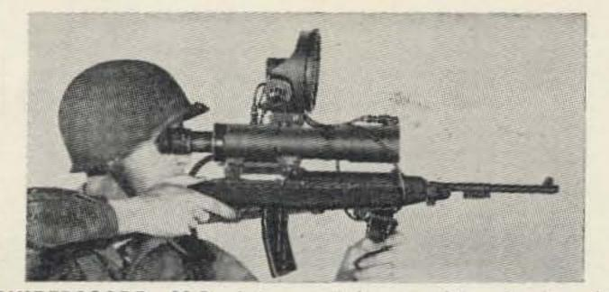
SNIPERSCOPE, M-3, late model, permits viewing in total darkness. Ready to use, includes 20,000 volt power supply. You furnish 6 volts DC to operate. Used, checked out. Rifle shown in picture not included.
