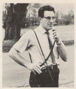
As a portable unit, the TR-22 operates from its own self-contained batteries. A carrying case and shoulder strap are provided with the unit, as is the pencil microphone with its curl cord. Power output is between 1.1 and 1.5W, depending on condition of batteries.
