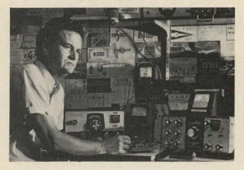
W B4SNC, Albert Coya, at his shack. The equipment is a HW -101 Heathkit, a HW 32 monobander for 20 meters, and a homebrew linear. Other gear shown homebrew phone patch, frequency counter, keyer, SW R meter, monitor scope, and power "Break, break, this is WB4SNC in Miami, looking for Nicaragua – is Nicaragua on the frequency, please?" I said in Spanish.
