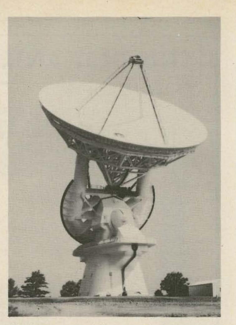
The largest equatorially mounted telescope in the world (optical or radio) is the 140 ft dish operated by the NRAO at Green Bank, West
