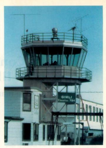
The Gimli control tower. The  $4 \times 6$ -element yagi for 2 meters is seen to the right and the 432-MHz beam can be seen to the left.
