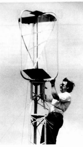
The helius rotor kit by Thermax for low-cost wind power.
