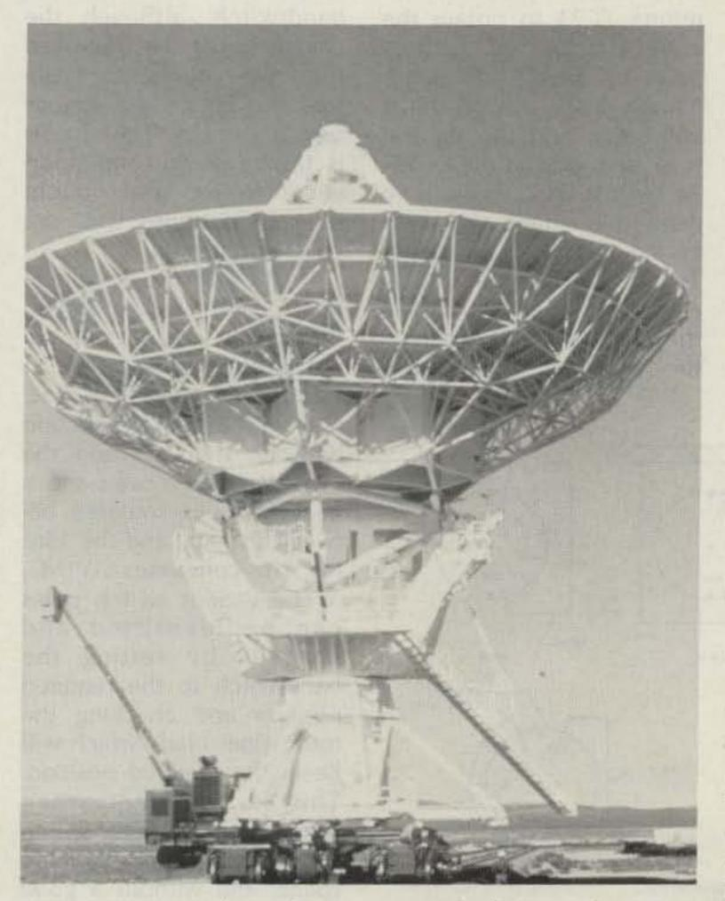
VLA antenna on the rail transporter which is used to move the antennas from one site to another.
