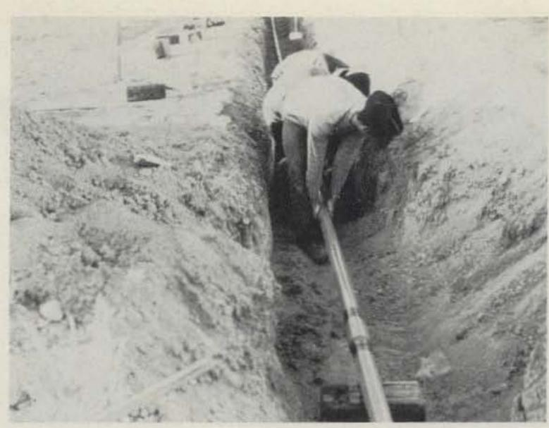
Installation of a VLA waveguide. These two-inch copper tubes serve as two-way communication channels. Control signals flow from the control building to the antennas in one direction, and the data from the observations flow in the opposite direction.
