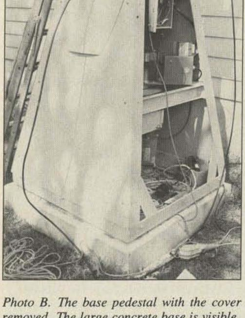
removed. The large concrete base is visible, as is the lazy-susan turntable at the top. (Photo by KT2B.)
