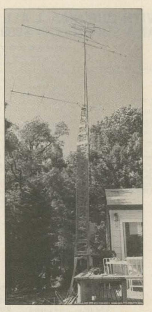
in an extremely strong support. The 256-lb., 28-foot mast could now support two climbers to allow antenna work in any tower position, up or down. I could remove the mast if needed by lifting it out with a ginpole or small crane.
