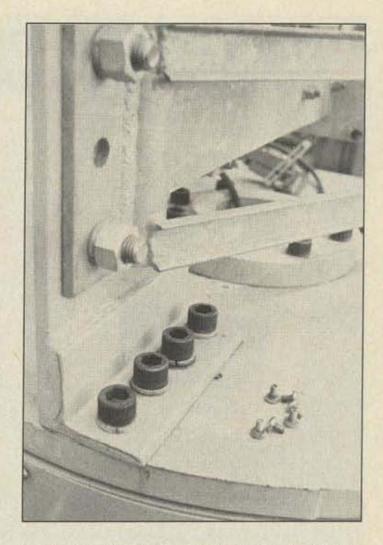
Photo C. Close-up of the method used to attach the tower to the rotating plate. (Photo by KT2B.)
