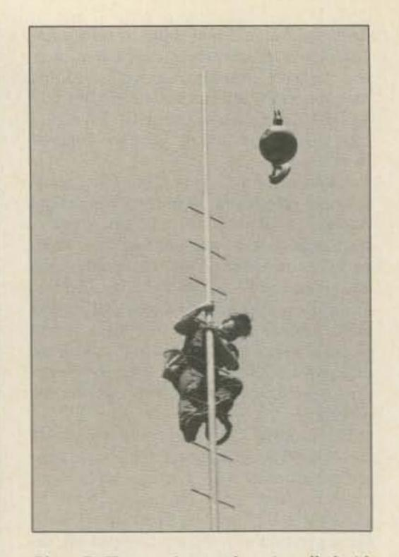
Photo E. The mast has just been installed with the help of a crane. WA2VUN is standing on Rebar steps. (Photo by WB2WIK.)
