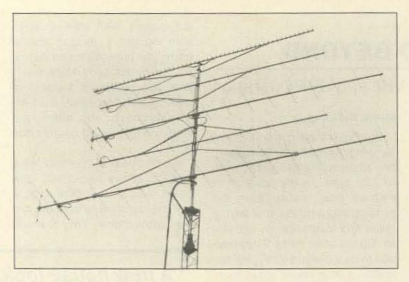
Photo B. Close-up of the 2m-23cm arrays on the W-51 tower.
