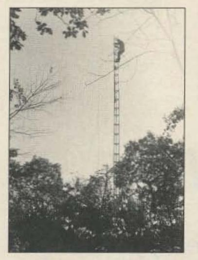
Photo B. Dave Porter K2BPP atop the 40-ft level, getting ready to put up the last 10-ft tower section.
