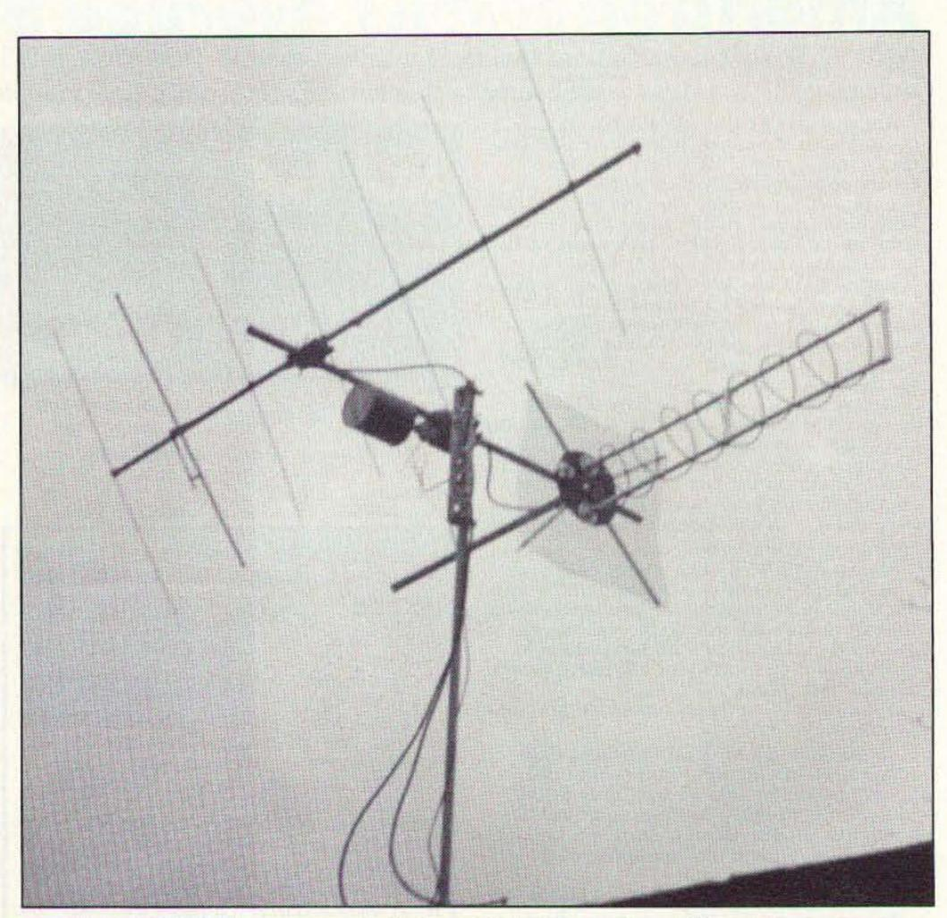
Photo A. K4OND's remote-controled rotating 2-meter yagi and 70 cm heilx antennas.
