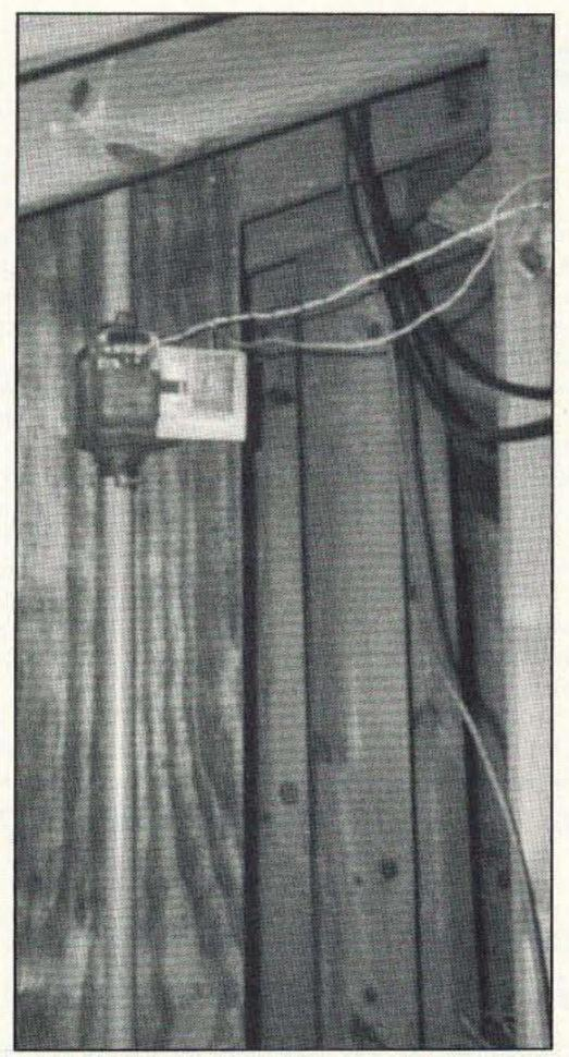
Photo B. The azimuth rotator is mounted between the rafters and the ceiling joists.
