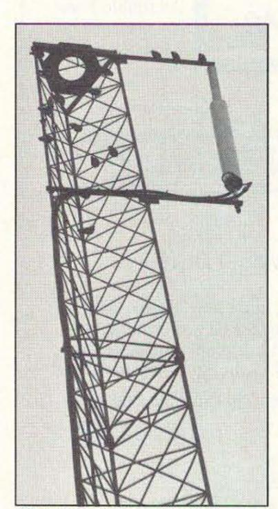
Photo B. Two Alford slot antennas (one for 439.25 and one for 910.25 MHz) are stacked on top of each other and side-mounted on the tower. Birds just love it! (Photo by Jim Pliett K9OMA).
