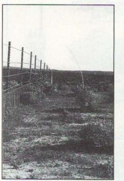
Photo B. Special fences along highways in California's Mojave desert keep tortoises off the road, where death would be almost certain. The white PVC pipe marks part of the survey grid.
