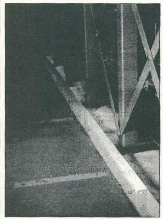
Photo E. These batteries have a spill pan and acid neutralized material on the floor. If you have a large system, this may be a local requirement — be sure to check!
