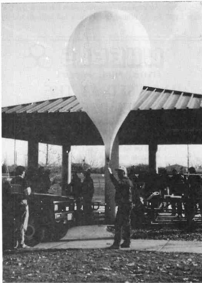
On the morning of May 11th, 1991, the balloon was inflated in preparation for liftoff. A bit of a breeze caused the balloon to move around quite a bit, so a large plastic sheet was used as a windbreak. The sheet was placed over the balloon to control it as it was carried over to the launch site. The balloon was raised, one last check of the payload and LIFTOFF!
