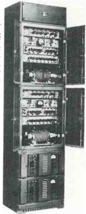
One rack of Microwave Receiving-Transmitting Equipment . . . a la Moscow! This rack holds two "Trunk Units," each capable of receiving and transmitting 600 telephone conversations, or one television channel. Power supply units are on the bottom.
