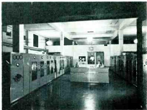
The Transmitter Hall of the British Broadcasting Corporation (BBC) shortwave station at Rampisham. The Hall contains 4 high-powered transmitters and was divided into two by a wall as a precaution during World War II.
