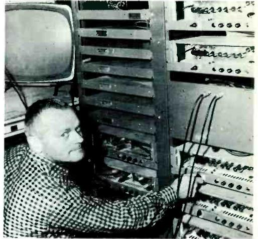
Making the many adjustments necessary at the "head end" of a multi-channel CATV installation.
