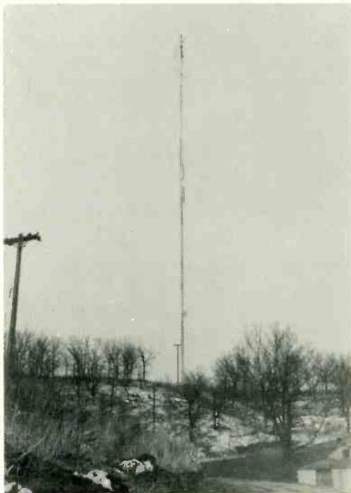
450 FEET ABOVE GROUND hidden in a swirling April snowstorm, the Redwood Falls, Minnesota receiving-transmitting tower looks anything but a "typical translator installation." Half way up—the transmitting antennas, at the top—the TACO ruggedized receiving yagis. Notes Klindworth, "I have over 400 TACO yagis in service, I've never had a major breakdown."
